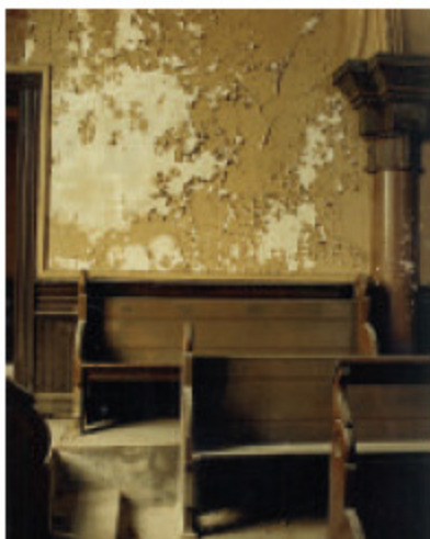
Eldridge Street Synagogue balcony, pre-restoration
