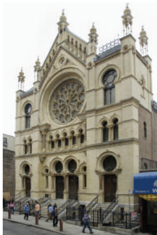
The Eldridge Street Synagogue opened in 1887; by 1900 many of its founding members had moved uptown.
