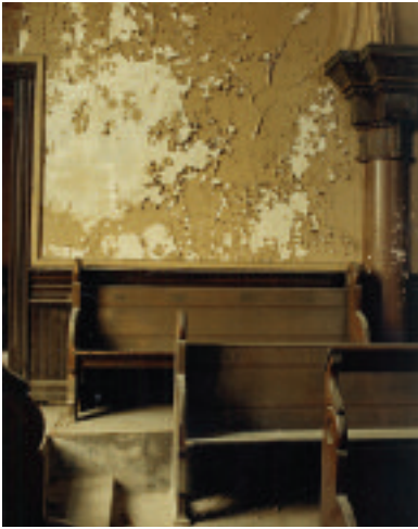
Eldridge Street Synagogue balcony, pre-restoration
